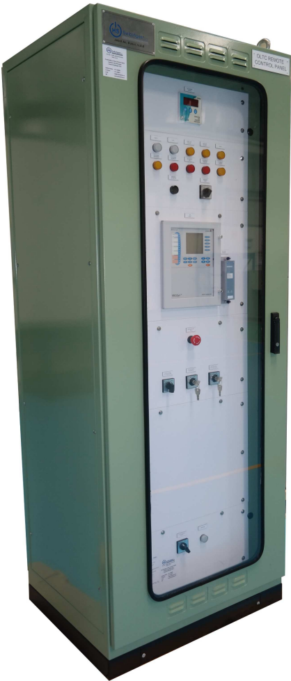
Control Protection Panel
